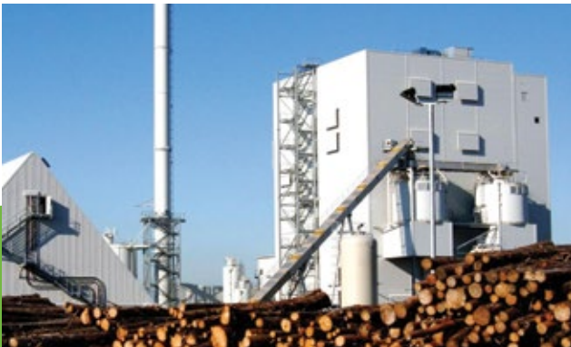
Biomass Power Station, Scotland
